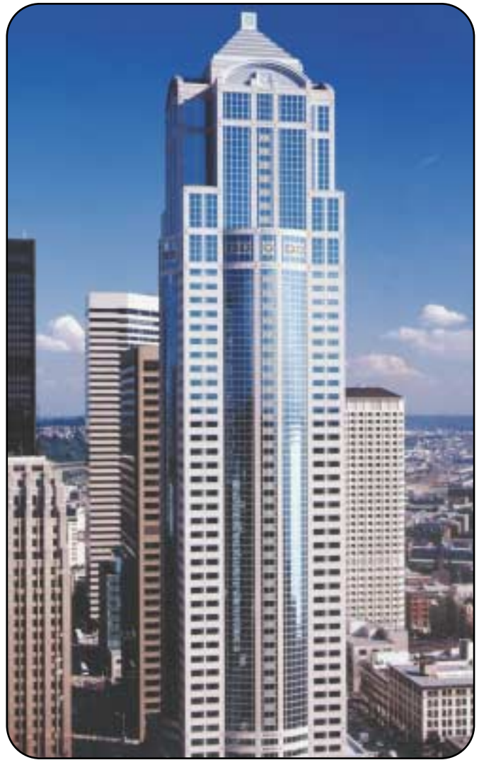
The asd's produced an immediate 66% demand reduction on the condenser pump motor and a 31% reduction on the chilled water pump motor at Seattle's Washington Mutual Tower.
