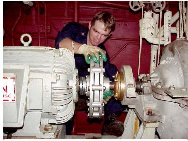
Navy seaman installs MagnaDrive Coupling on a seawater pump.
